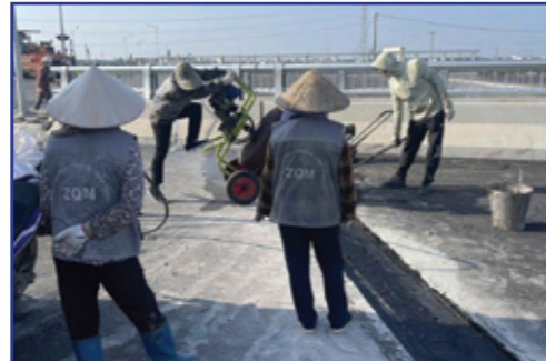
Khe FEBA – FEBA joint
